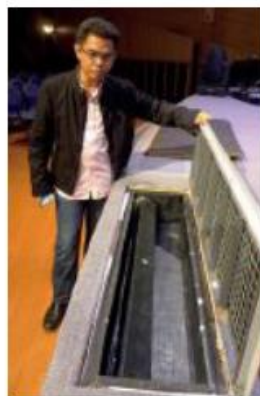
Church consultant Erwin Balangue reveals one of the four hidden K-Array KP102 speakers that serve as stage monitors
